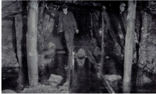
Figure 3: Water seepage in an abandoned mine during the miners' strike.
